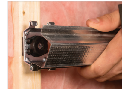
Engage Pliteq® Furring Channel into either claw, then squeeze channel to engage the claw
